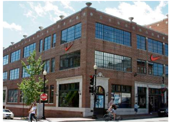
A three-story, 31,000 SF Nike retail store is adjacent to the Property.
