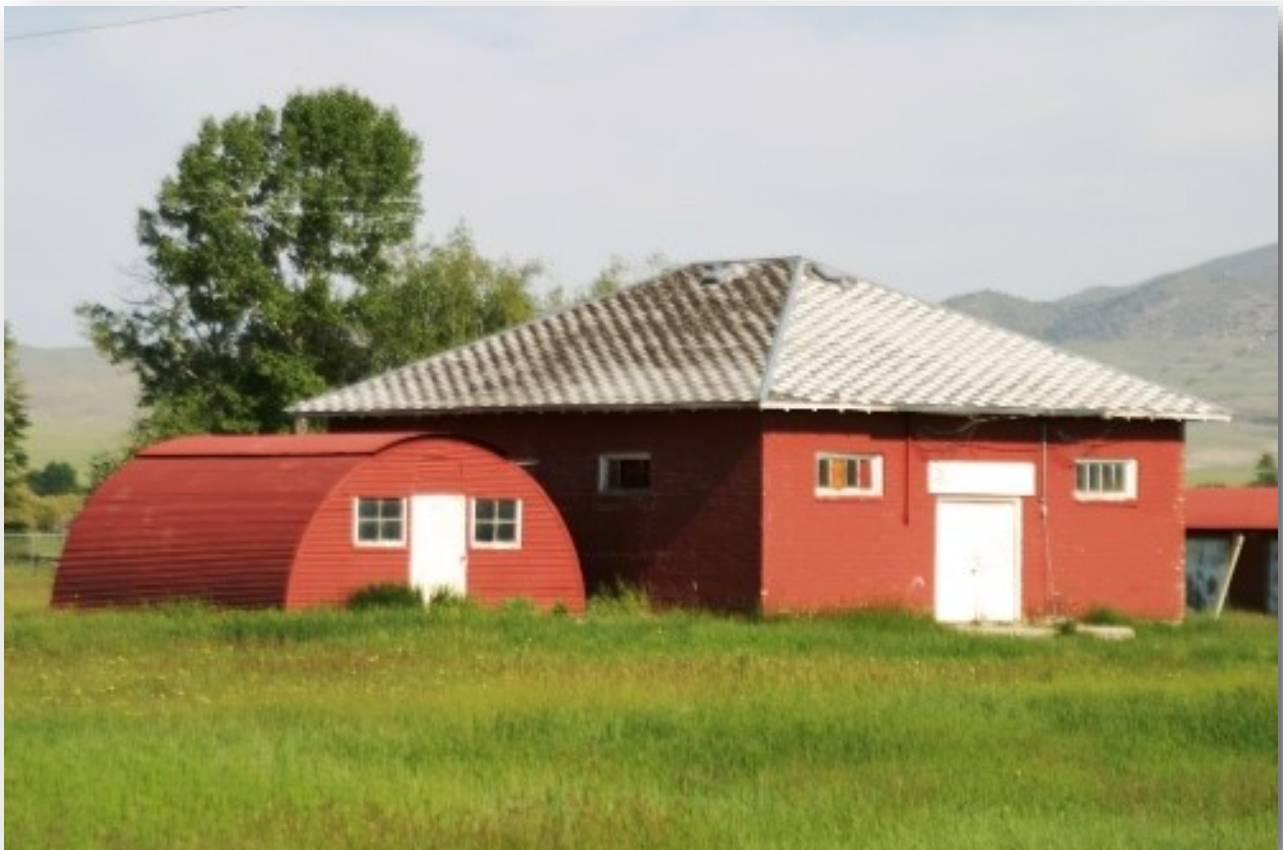
The Carpenters Shop
