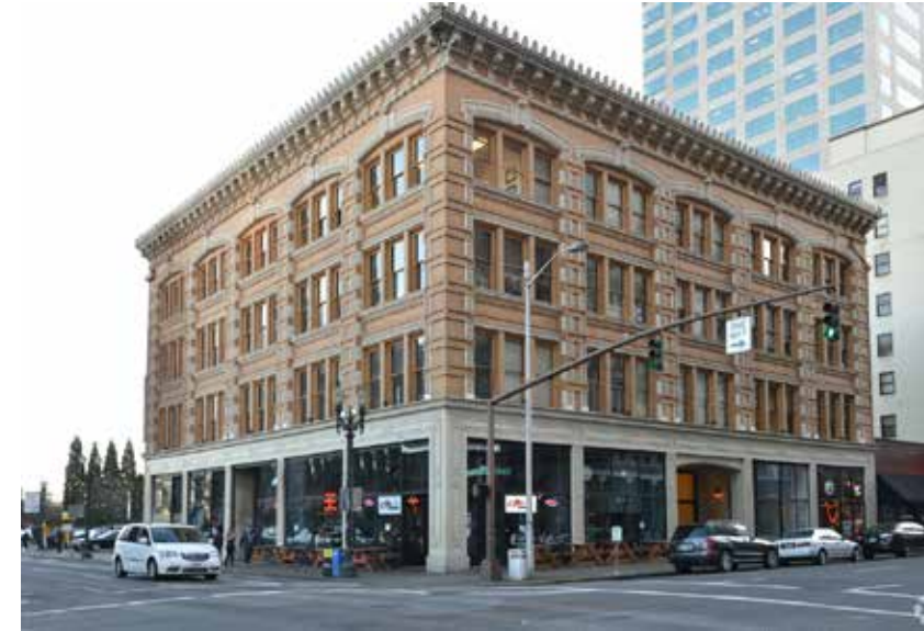
6 THE POSTAL BUILDING
