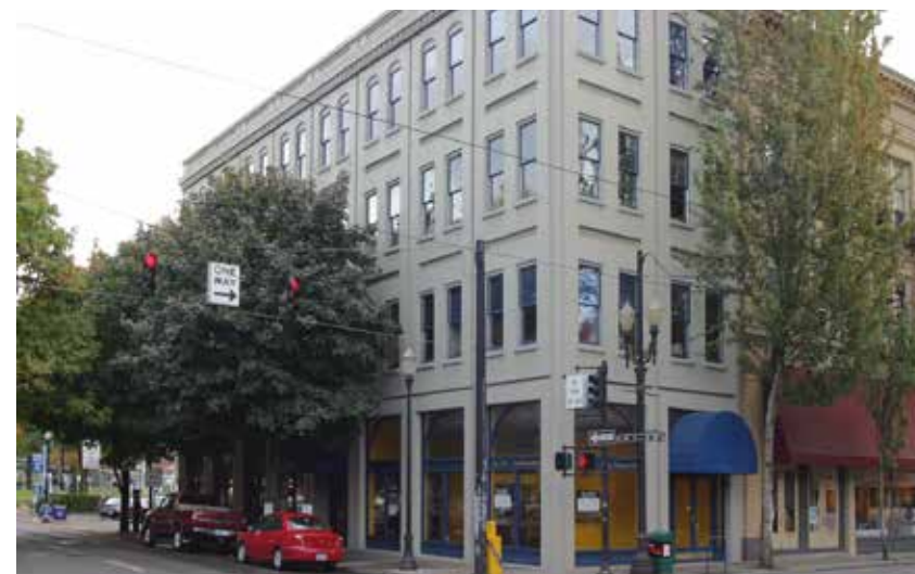
6 KAPPES MILLER BUILDING 50 SW Pine Street • Portland, OR 97204
