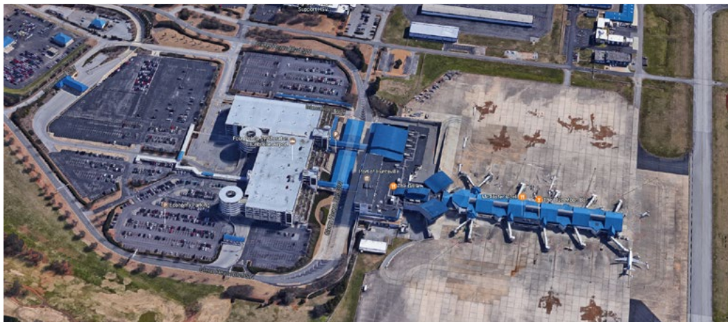
Huntsville International Airport
