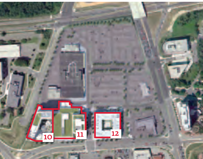
Phase 1 - Building 11 Completion: Summer 2014 80,000 SF Office
