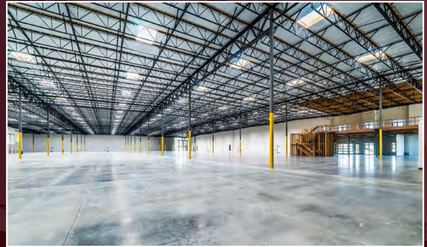
30' Clear Height Warehouse
