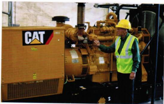
Green Carbon's Phil Wilson checks a control on Caterpillar's synthetic gas-powered generator that powers Green Carbon's Thermal Vacuum Reactors. (Photo courtesy of Doug Walker RN-T)
