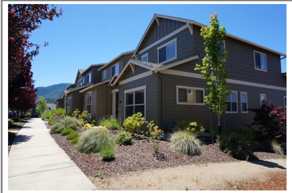
View of Camelot Drive townhomes located west of subject
