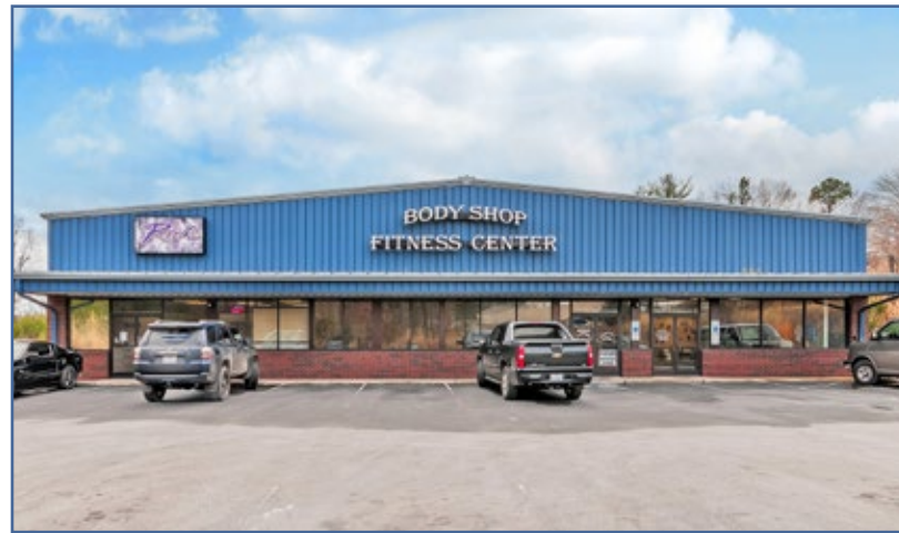
Front of building showing entrances for the two tenants
