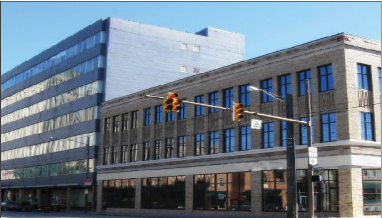
FRONT OF BUILDING
