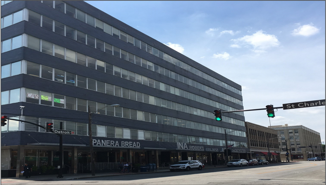
FRONT OF BUILDING
