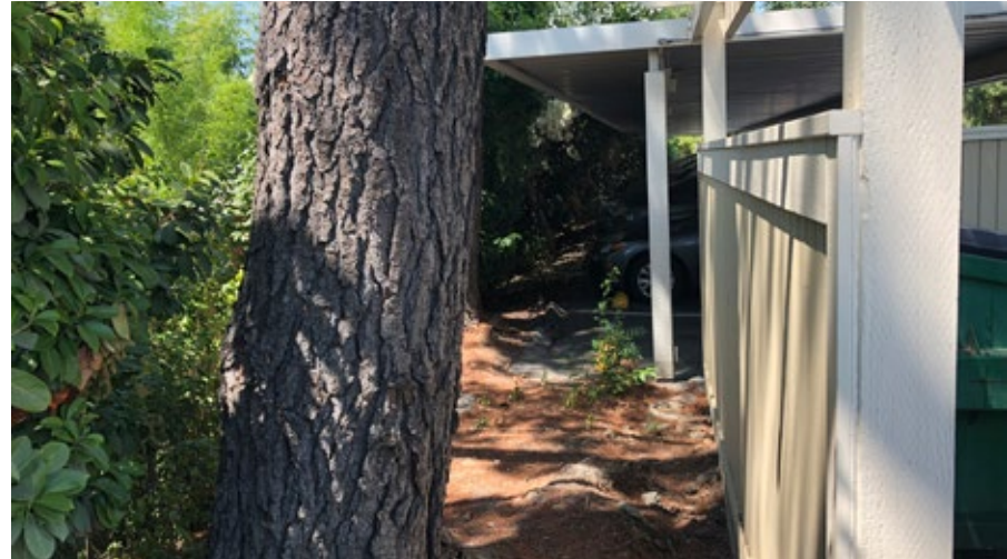
Adjacent Property Edge (Looking North)
