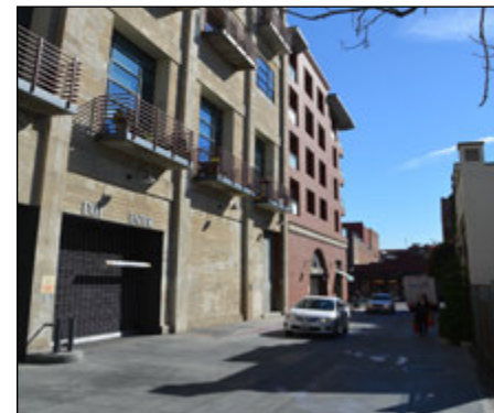
Parking Structure Access
