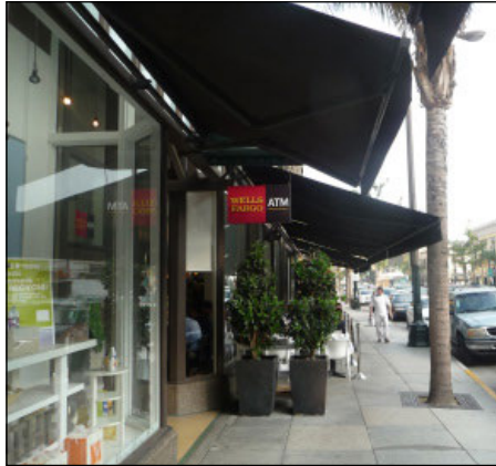
Retractable Awnings to provide shade during appropriate times of year or day
