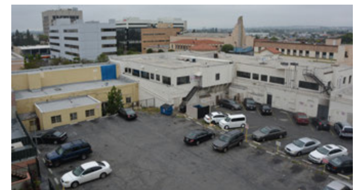
Examples of vacant areas with potential for development behind Market Street shopfronts
