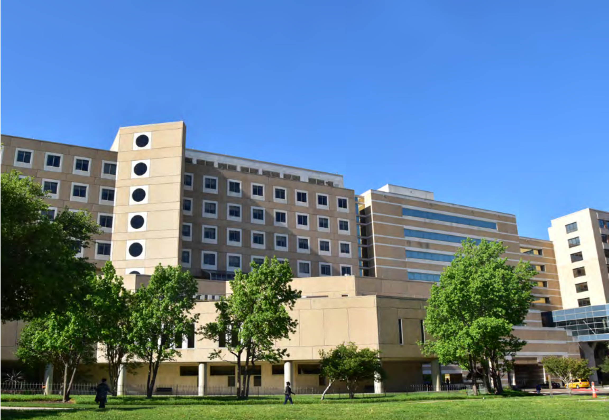
From left to right: Zale Lipshy Hospital, Charles Cameron Sprague Clinical Science Building, and Old Parkland Hospital
